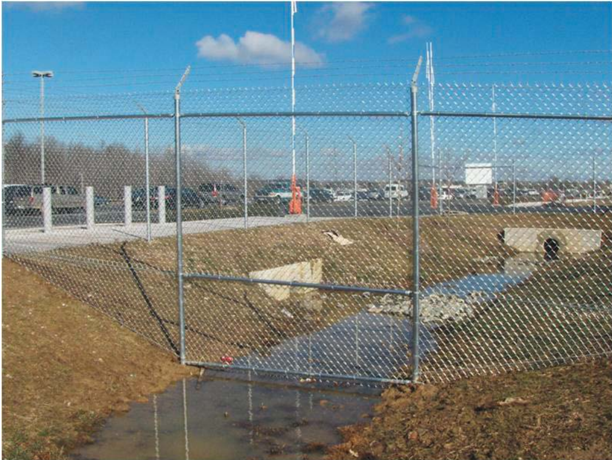
Figure 14 Chain link fence over ditch
