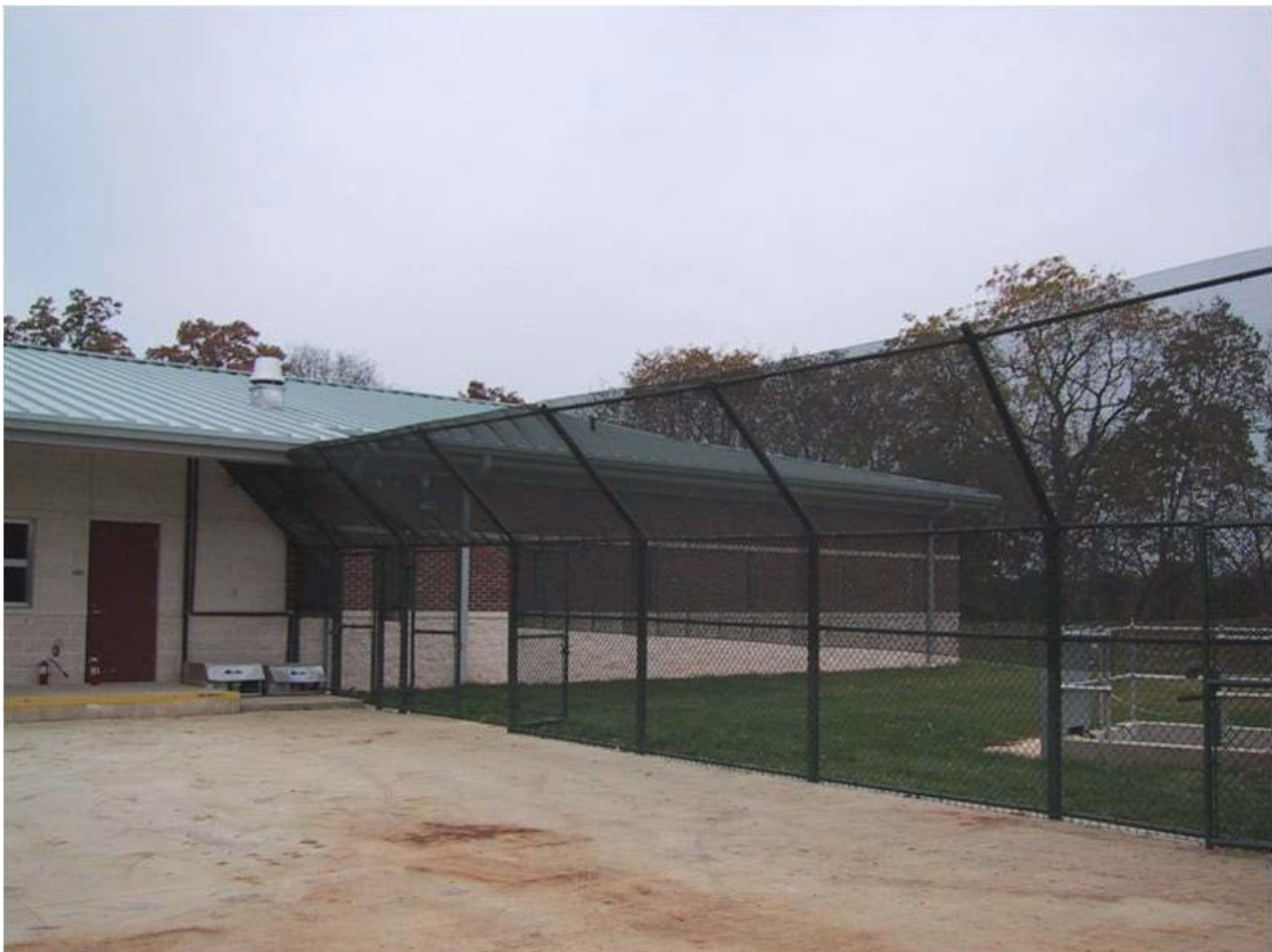
Figure 5 Welded wire mesh fence
